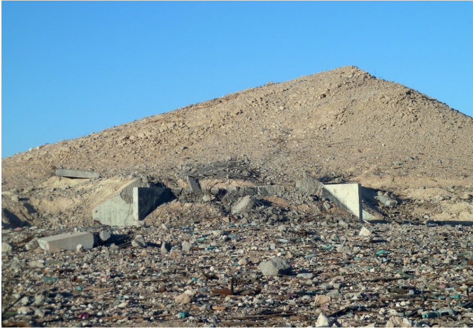
Chart 6: Explosive store house destroyed by NATO air attack, Libya, 2011
